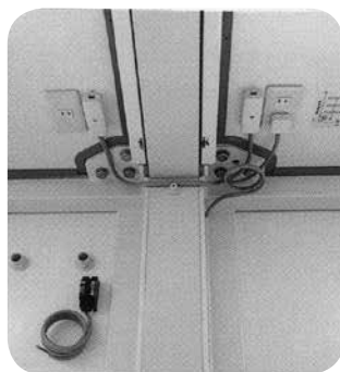
連棟部入電側
